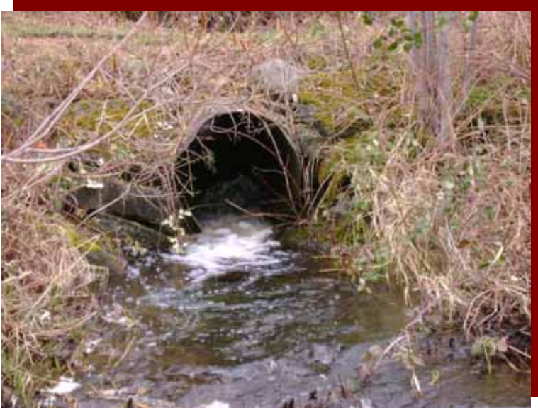
Old culvert with no bottom
