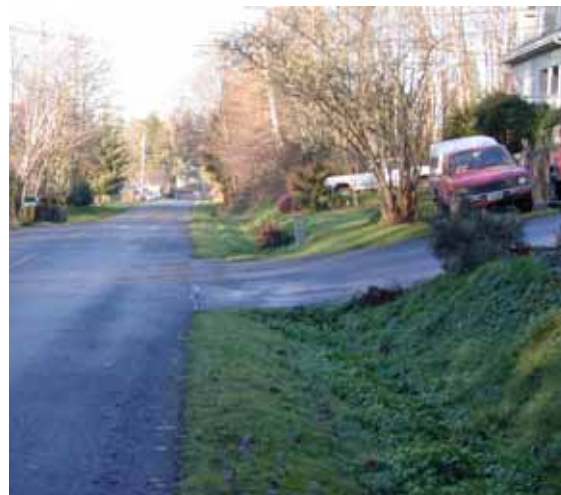
Typical roadside ditch and culvert system in South Warm Beach residential area (Clarence Ave)
