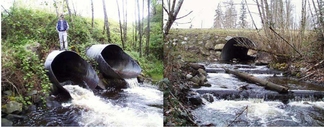
French Creek before and after a culvert replacement
