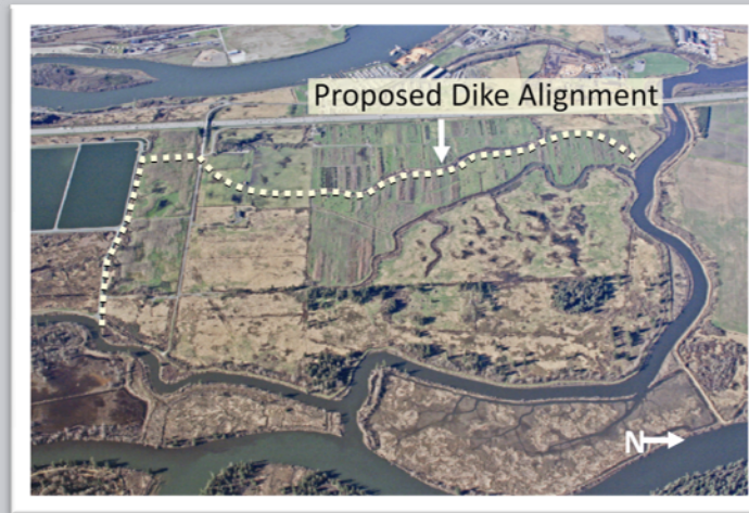
View of project area looking west showing the proposed dike alignment (approximate). The City of Everett wastewater treatment facility is in the upper left of the photo to the south, I-5 parallels the project area to the west, and Union Slough encircles the project area to the north and east.
