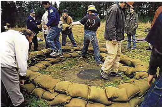
Washington Conservation Corps members learn how to build a ring dike.
