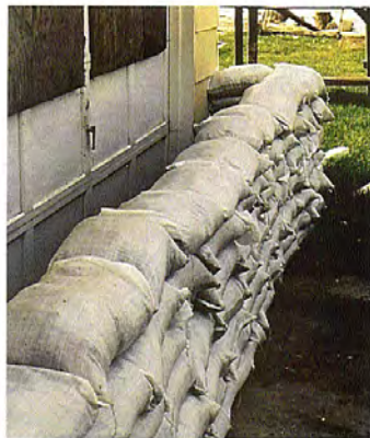
Single stack placement
