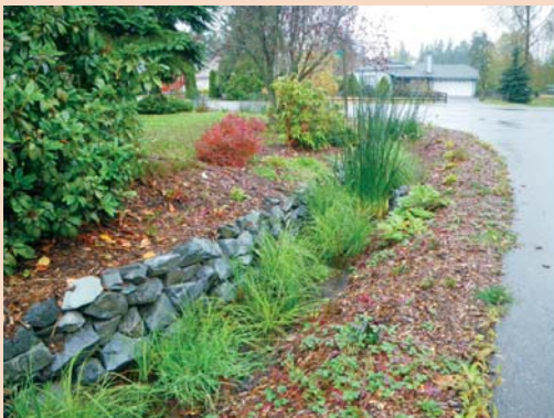
Natural Drainage Project: Roadside Ditch Enhanced with Rain Garden.
