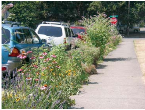
Natural Drainage Project: Parkway Enhanced with Rain Garden Strip.
