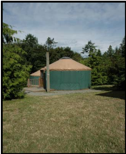
Figure 4: This yurt at Kayak Point should be part of an inventory with maintenance requirements and condition for each asset.
