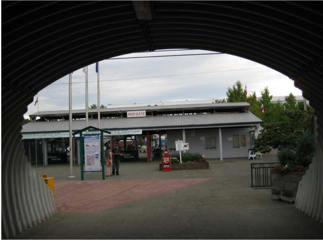
West pass gate and ticket booth viewed through pedestrian tunnel
