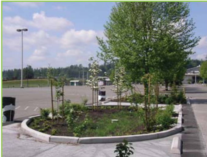
This bioswale is one of the many examples of low impact development (LID) best practices installed as part of an LID demonstration project at the Evergreen State Fairgrounds.
