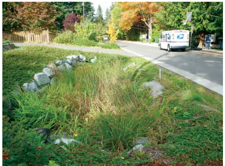
Vegetation planted in swale to filter out pollutants
