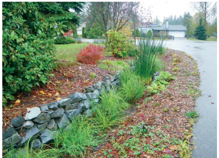
Rain garden installed in place of roadway shoulder
