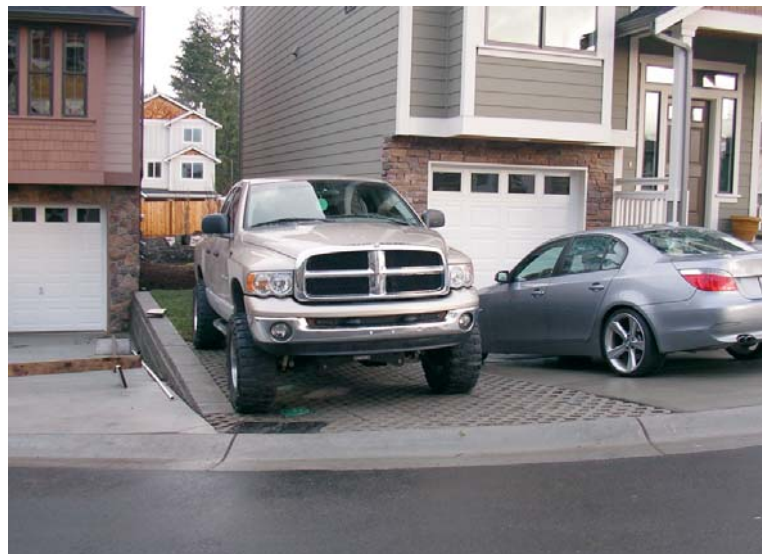
Pervious pavement at end of driveway
