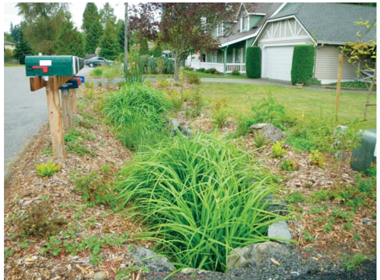
Vegetation planted in ditch to filter out pollutants
